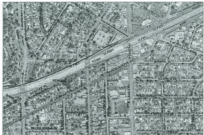
Water Mains - Park Avenue (Phase II)
