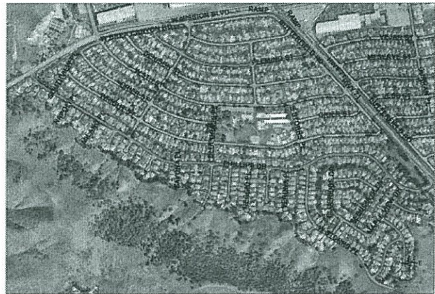
Water Service Replacement (Residential) - Westmont Area
