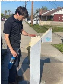
The Water Resources Department has water-sampling stations throughout the City's water distribution system. The purpose of these stations is to facilitate the collection of routine water quality samples. Every week, the water quality team collects individual water samples from 35 designated sample stations. Before collecting samples, staff conduct an onsite field analysis for pH, temperature, and chorine residuals.
