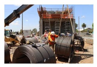
Just to the east of the bridge work, crews continue to construct the east approach, as seen in the photo below (left). Crews are currently constructing the retaining walls for the approach, which consist of custom form panels that feature the project's citrus design.
