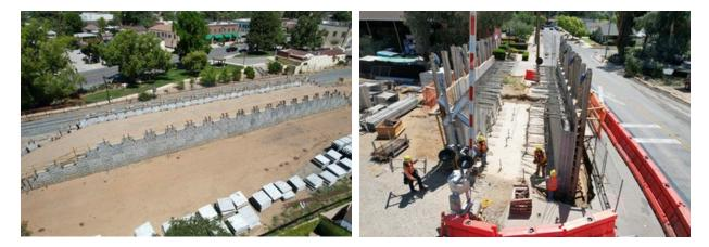
**Light Rail Track System:** Along the project corridor just north of Arrow Hwy. in San Dimas and La Verne, crews have begun constructing the foundation for the light rail track system by placing layers of subgrade, sub-ballast and ballast (crushed rocks) throughout the light rail track portion of the corridor. Crews will later install the light rail tracks on top of the ballast.
