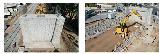
Across the intersection, the east approach for the bridge (photos above) continue to take shape as crews construct the retaining walls. The retaining walls for both approaches consist of custom form panels that feature the project's citrus design.
