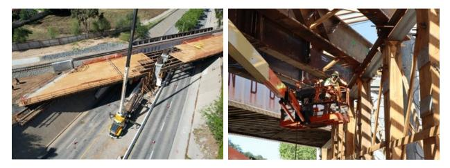
**Lone Hill Ave. Bridge (Glendora):** With the center columns and both abutments completed, crews are now focused on assembling and installing the falsework over Lone Hill Ave. The falsework is the temporary support for the super-structure as it is built across the street and is made up of a combination of steel and wood beams. Crews are currently assembling the parts for the falsework onsite (photos below). Once in place, the falsework will span from abutment to abutment.
