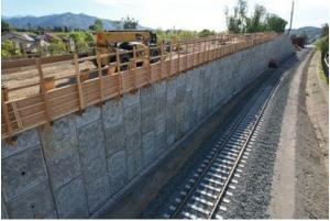
Additionally, work continues on the west approach, as seen in the photo above (right), which has been under construction since last summer. Across the intersection, the east approach for the bridge (photo above) is now starting to take shape as crews construct the retaining walls. The retaining walls for both approaches consist of custom form panels that feature the project's citrus design.
