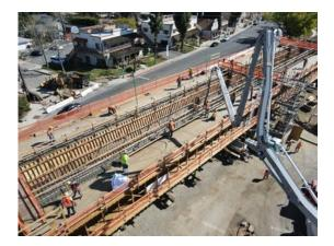
Crews have also begun constructing the west approach (photo below, left) for the bridge. The west approach will measure approximately 400 feet in length and consist of custom form panels that feature the project's citrus design. The length of the east approach means that the railroad crossing at Monte Vista Ave. will later be permanently closed to vehicular traffic. Pedestrians will be able to travel north and south on Monte Vista Ave. by way of a pedestrian undercrossing (photo, below right).
