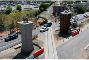
The Lone Hill Ave. bridge will be the largest bridge on the 9.1-mile project from Glendora to Pomona. When completed, the bridge will span 344 feet from abutment to abutment. The super-structure will have a minimum vertical clearance of 24 feet to allow freight trains to travel underneath. This is the one location between Glendora and Pomona where the freight system will switch from south to north positions in the corridor to continue serving customers.
