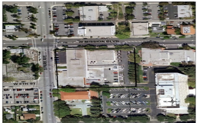
Police - Main Facility Roof Replacement
