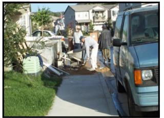
Don't hose down the pavement. Do use a broom to clean up spilled materials
